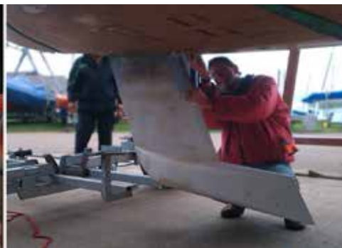
Exposed keel was cleaned, epoxied and reinstalled
